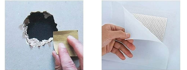
1. Lightly sand around hole and wipe clean 2. Tear off the sticker
